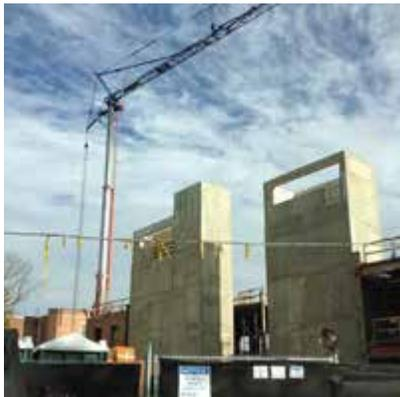
Construction continues of the future site of the new Fellowship Building, at 1700 Wisconsin Avenue. This month saw the erection of two enormous elevator shafts, extending well above the building's profile, as well as the arrival of the crane. The building is scheduled to open its doors in the fall of 2014.
